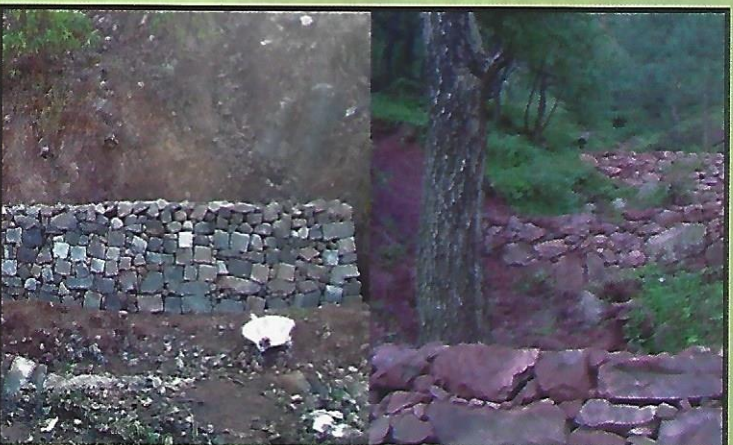
Check Dams in Dry Rubble Stone Masonry constructed in Co. 18/Blr of Billawar Range of Billawar Forest Division
